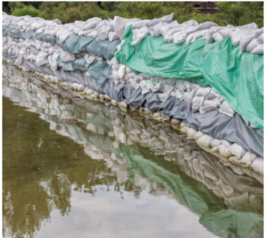
A temporary wall of sandbags to prevent flooding
